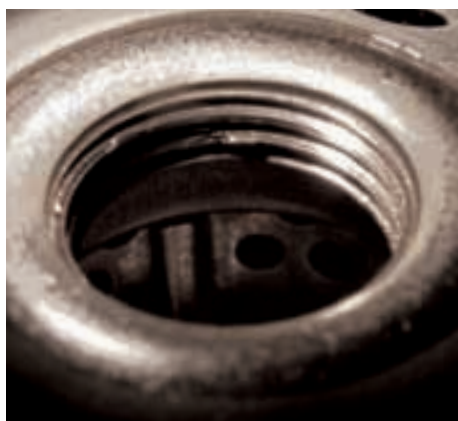
Fig. 5 Damaged threads due to an incorrectly installed filter
